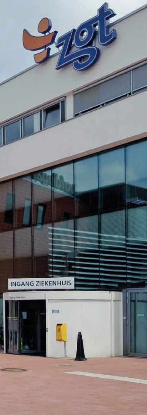
Ziekenhuisgroep Twente (ZGT) comprises two hospitals in Almelo and Hengelo (photo). Siemens not only assumes full responsibility for the quality and uptime of imaging systems, but also ownership.
