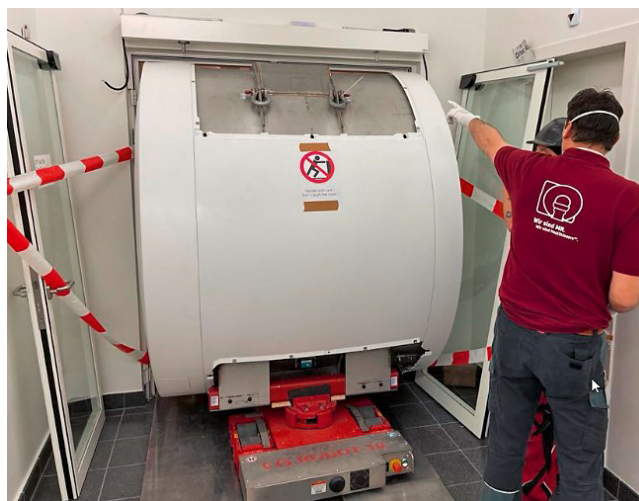
5 MAGNETOM Free.Max installation at University Hospital Basel in Switzerland. Even during one of the very first installations, the small size of the system and the eliminated quench pipe paid off to make the installation process much easier.
