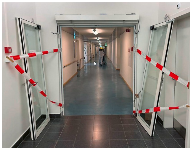
5 MAGNETOM Free.Max installation at University Hospital Basel in Switzerland. Even during one of the very first installations, the small size of the system and the eliminated quench pipe paid off to make the installation process much easier.
