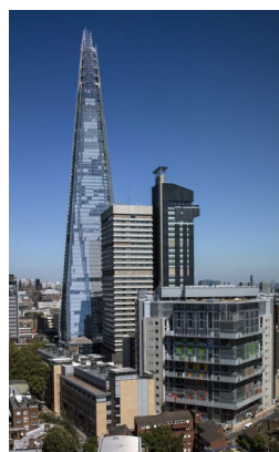
King's College London and Guy's & St Thomas' PET Centre, UK. (Left) St Thomas' Hospital (Right) Guy's Hospital.
