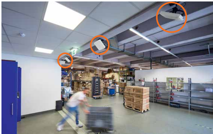
The container of empty packaging is taken from the goods elevator. RFID antennas read the entire contents of the container.
