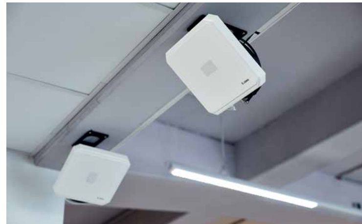
The container of empty packaging is taken from the goods elevator. RFID antennas read the entire contents of the container.
