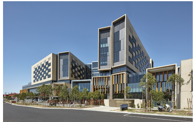
Bendigo Hospital Project, Australia
