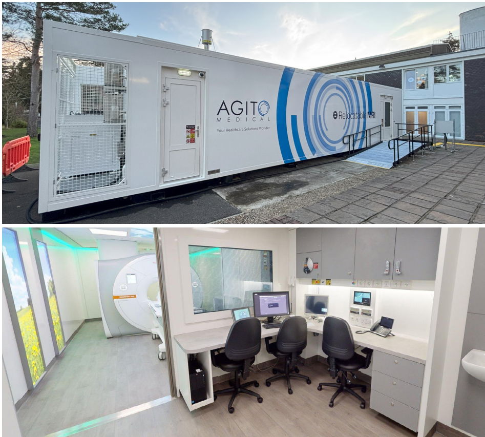
2 A 1.5T MAGNETOM Sola deployed in a relocatable unit in the UK.
